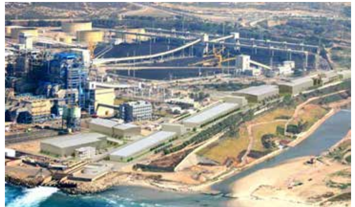
The Hadera Desalination Plant on the Mediterranean Sea, 28 miles south of Haifa, which opened in December 2009. It was designed so that it can function as two separate plants, operated independently.
