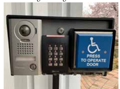
Key volunteers and staff use individually coded plastic fobs with the keyless entry pad at TI’s front entrance.
